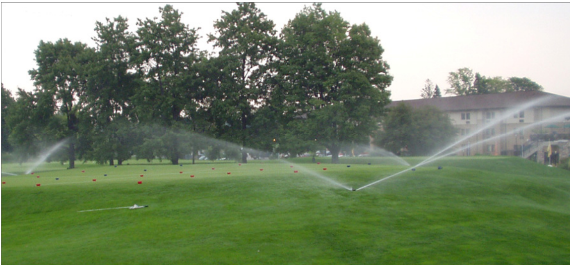
Figure 2. Sprinklers in operation during audit
